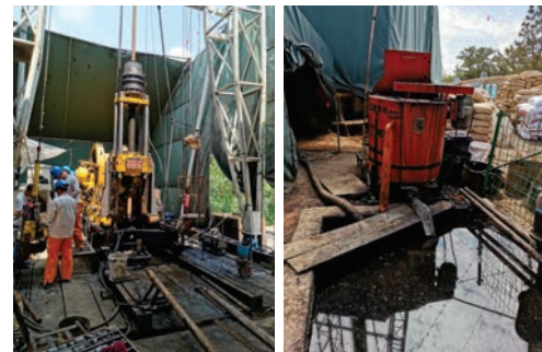
(a) Drilling rig (b) Mud pit
