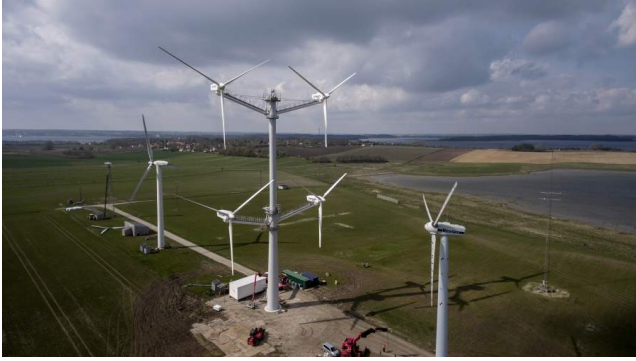
Fig. 1. Vestas MRT demonstrator, consisting of 4 V29 225 kW nacelles and rotors. Courtesy of Vestas Wind Systems A/S.
