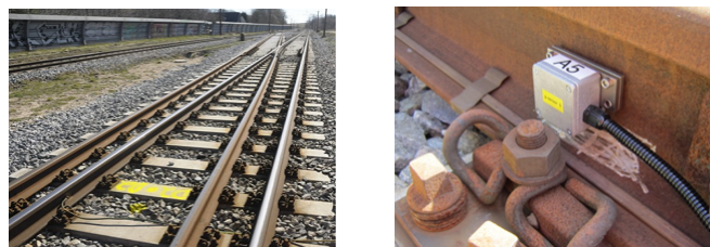
(a) Overview of the turnout
