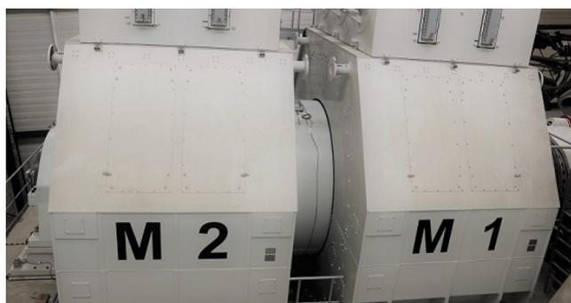
Fig. 2. Synchronous drives coupled with a tandem shaft
