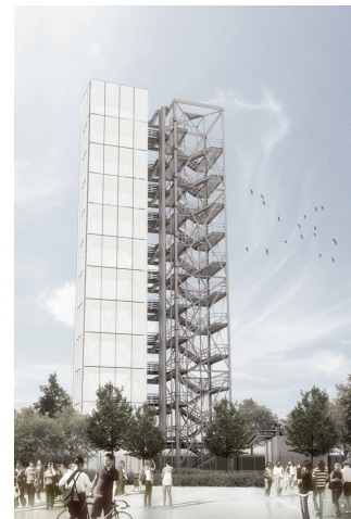
Fig. 1. Rendering of the high-rise adaptive truss structure with access tower at the Campus of the University of Stuttgart, Germany. Source: ILEK, University of Stuttgart
