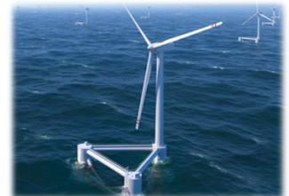
One of the primary difficulties of this approach is controls-related: the floating system is more dynamic and potentially closed-loop unstable. Wind turbine controllers must now, on top of their existing objectives of power production and load regulation, avoid large platform oscillations and accommodate wave disturbances. We invite papers which examine solutions to this complicated problem.
