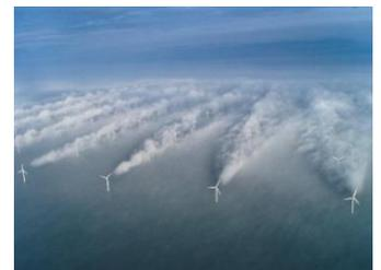
shown that because of this interaction, control strategies that are optimal for individual turbines can be sub-optimal at the wind farm level. Designing a wind farm controller, or turbine-to-turbine distributed control strategy, which can outperform individual turbine only control is the focus of research at several centers.
